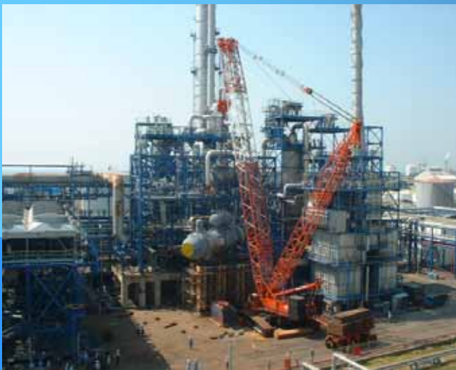
Replacement for Heat Exchanger
