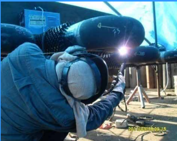
U – Bend Tube Welding
