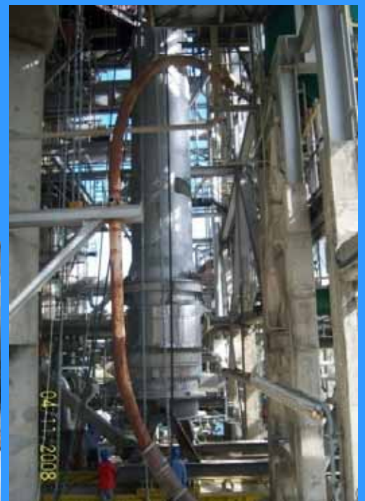
Replacement for Catalyst Cooler
