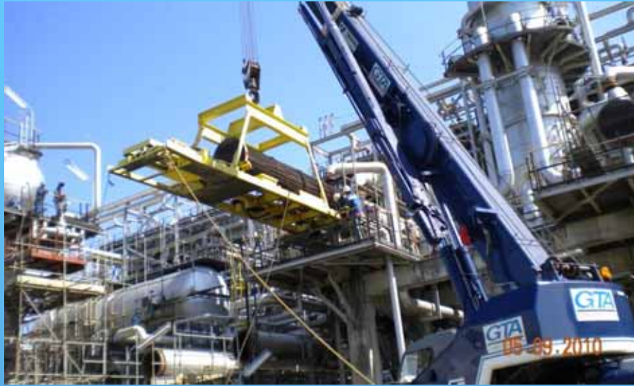
Cleaning & Repair for Heat Exchanger Tube-Bundles
