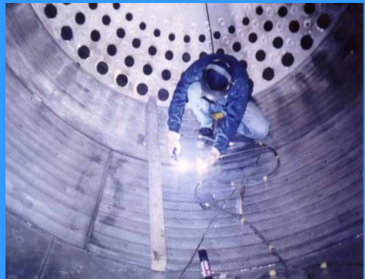
Repair for Shell of Dryer
