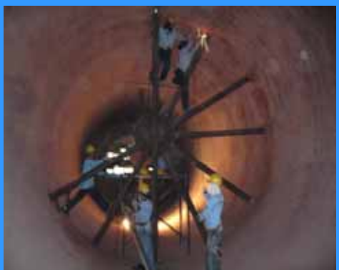
Welding Shell Kiln
