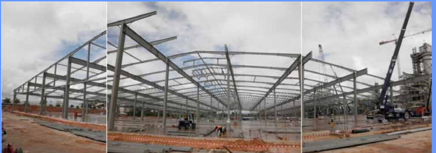
Assembling and Installation for Building Steel Structure
