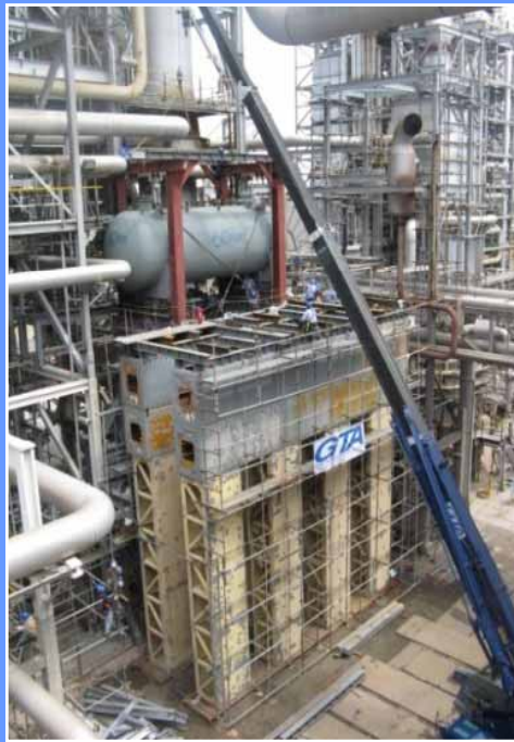
Installation of Drum for Revamping Work
