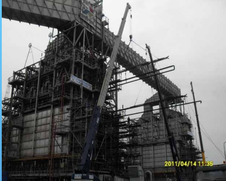
Re-tubing for Oil Refinery Furnace Radiant & Convection Tubes
