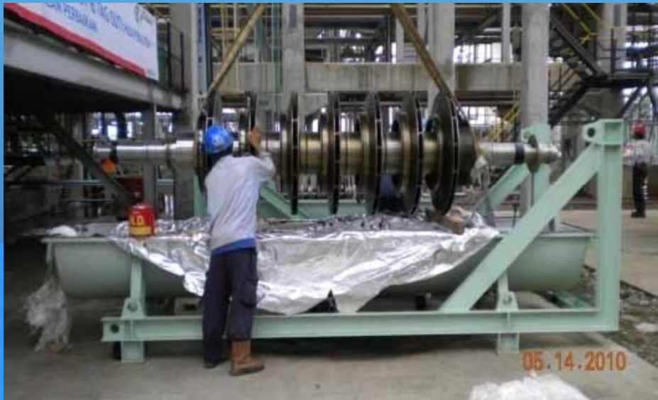
Over Haul for Turbine Compressor
