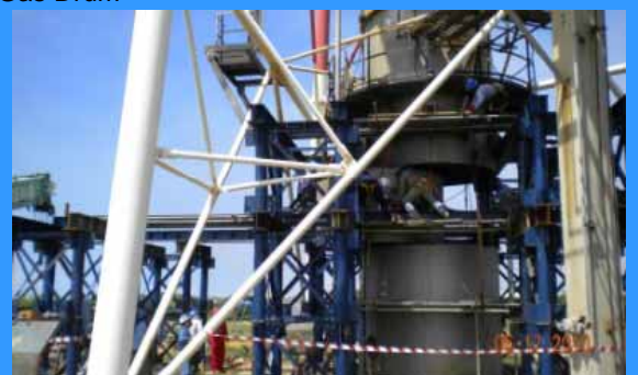
Replacement for Flare Shell Gas Drum
