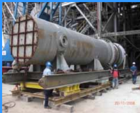
Replacement for Catalyst Cooler
