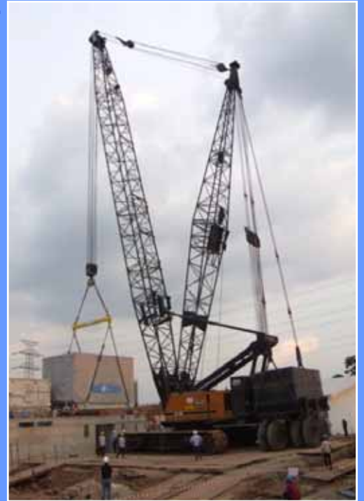
Installation for Turbine Generator
