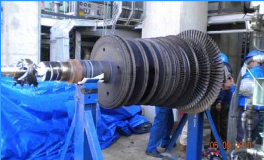
Over Haul for Turbine Compressor
