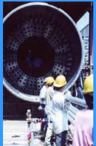
Re-tubing for Dryer's Tubes
