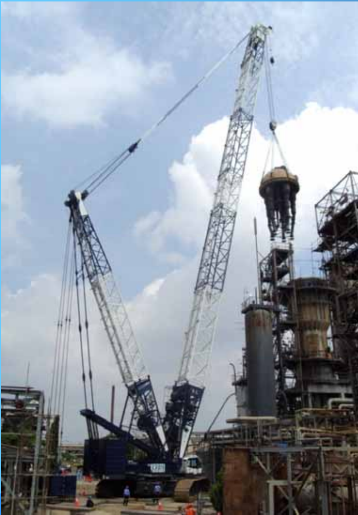
Cuting Shell Top Regenerator and Lift Down the Cover Include Cyclone Unit
