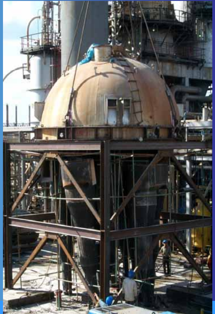
Repair for Planum of Regenerator
