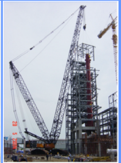
Assembling and Installation for Steel Structure by Module Method
