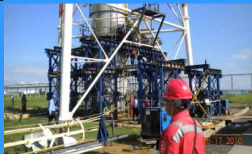
Replacement for Flare Shell Gas Drum
