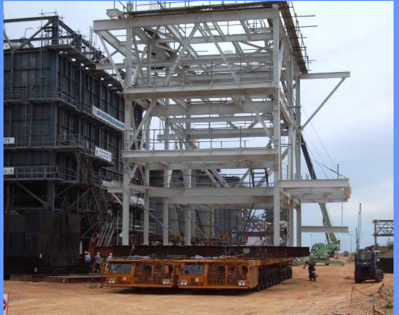
Transportation for CCR Structure
