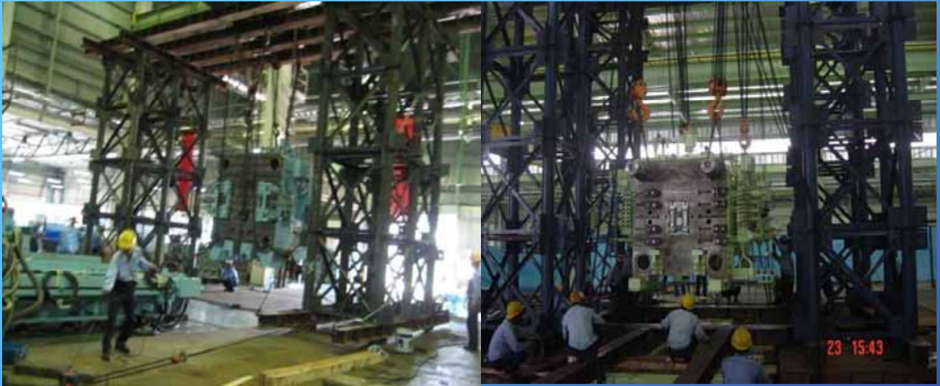
Installation for 1,250 Ton Die Casting Press Machine
