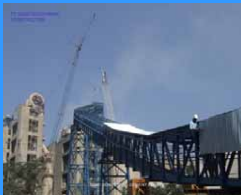
Installation for Siding Conveyor
