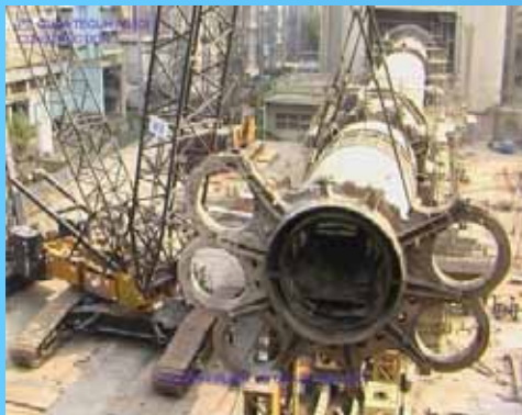
Installation for Shell Kiln
