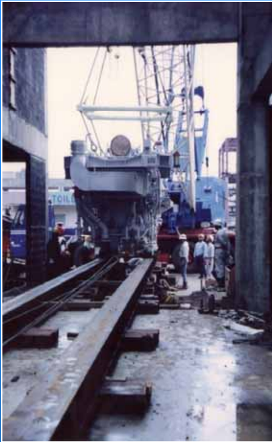
Installation for Engine Generator
