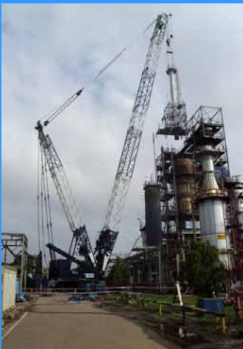
Replacement for Regenerator Stack
