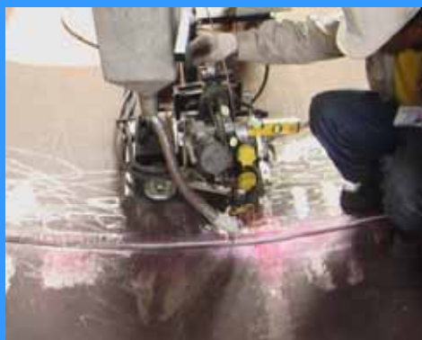
Welding Shell Kiln
