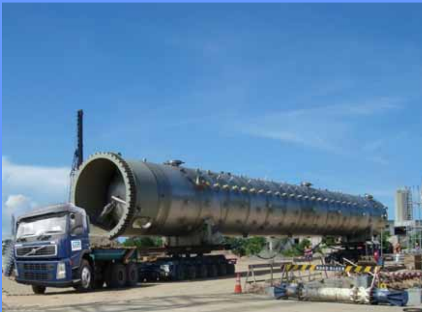
Transportation for Absorption Tower
