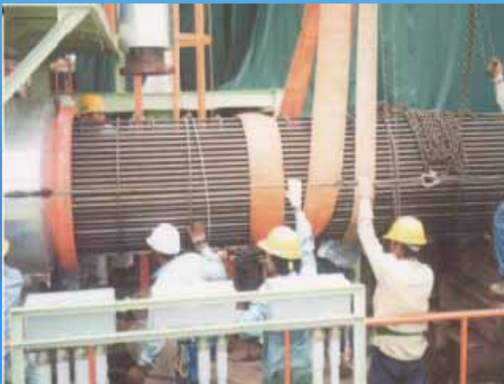
Cleaning & Repair for Heat Exchanger Tube-Bundles
