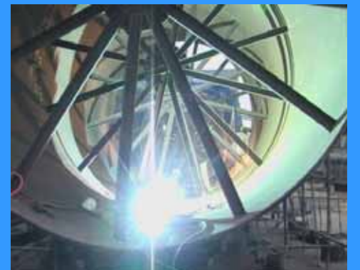
Welding Shell Kiln
