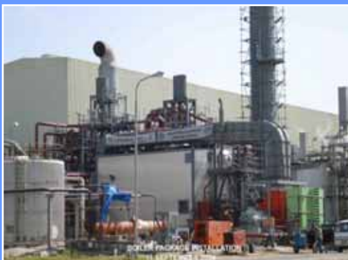
Installation for Boiler Package
